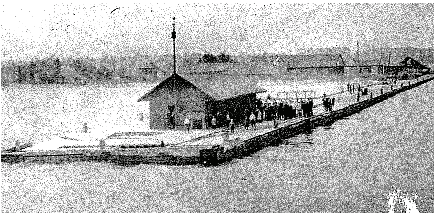
Oshawa Harbour, west wharf with storage elevators in the background.
